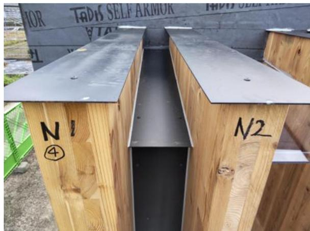
[図. 調査箇所④上部-鋼製笠木周辺部・CLT1-CLT2 (例：北面)]
