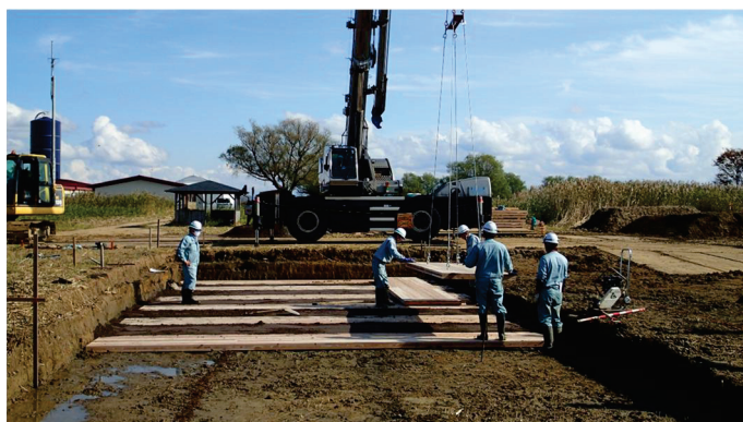
(c)CLT の敷設状況
