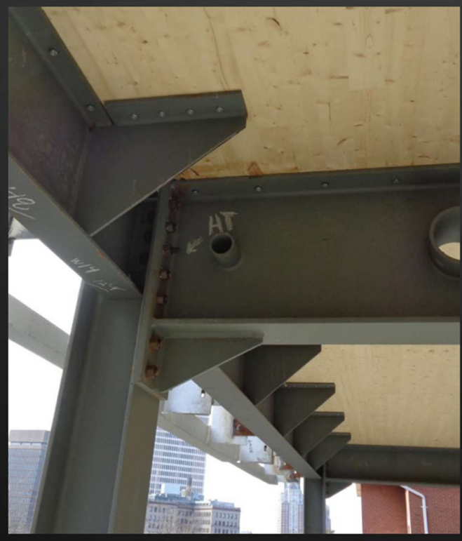
Weak Axis Column Bracing at Floors
