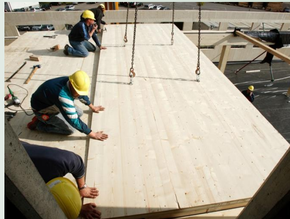
assembling of ceiling elements
