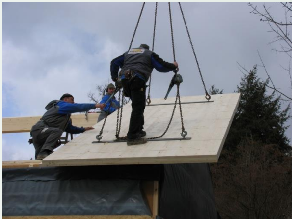
assembling of roof elements
