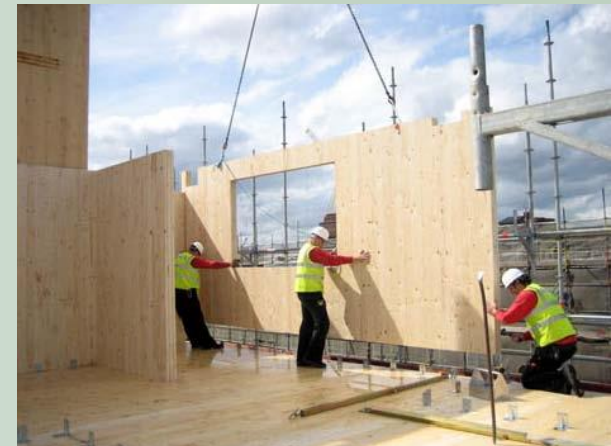
assembling of wall elements
