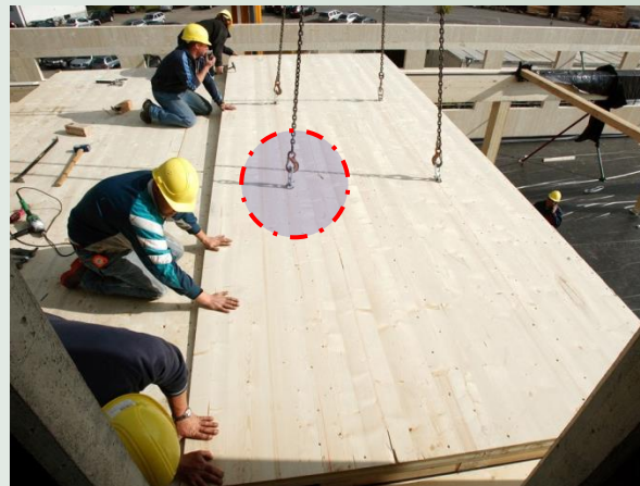
mounting parts for ceiling elements
