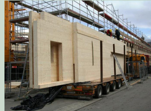
discharging (building site)
