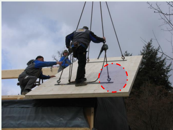
mounting parts for roof elements
