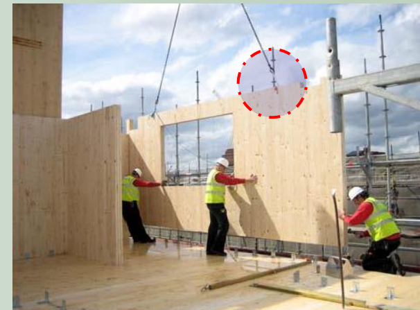
mounting parts for wall elements
