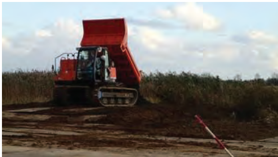
(c) 掘削土の運搬
